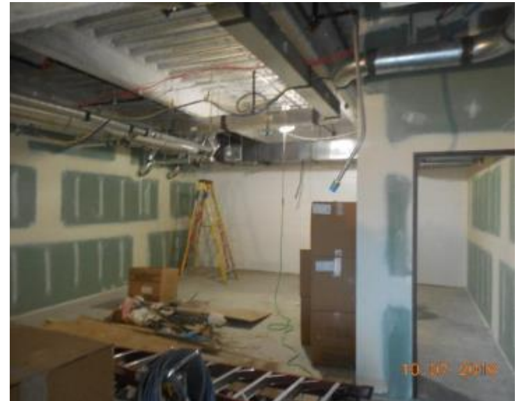
Kitchen Area in Progress
