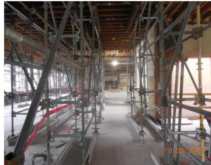
Shoring in Historic Building
