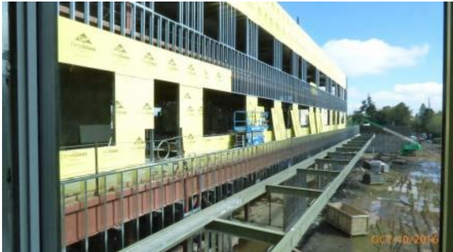
Exterior Walls Ongoing
