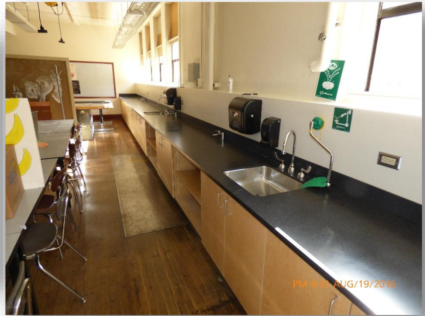
MLC 2 New Science Classroom Upgrades
