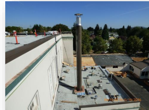
Sellwood MS New Chimney Stack
