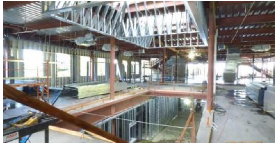
Interior Wall Framing Prep
