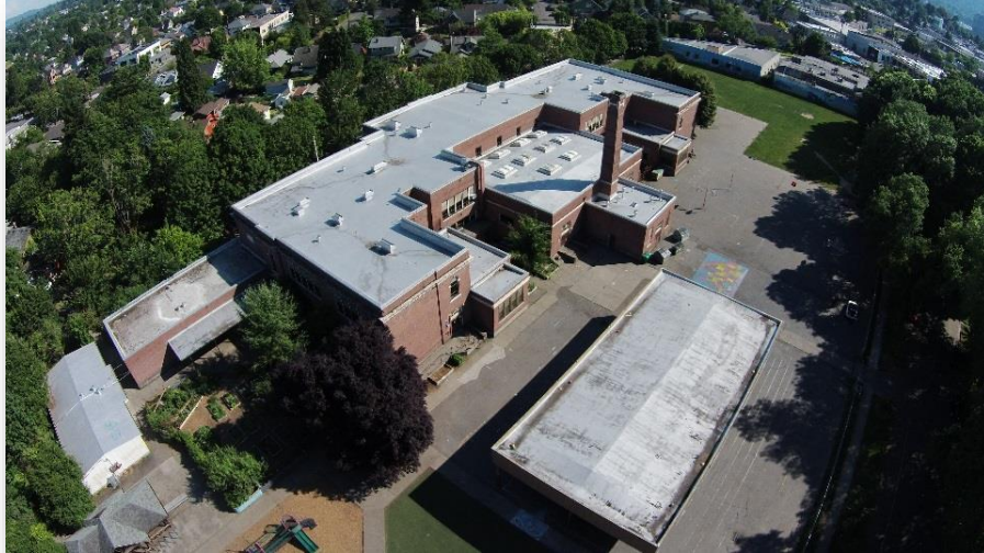
Abernethy 29,000 SF of New Roofing
