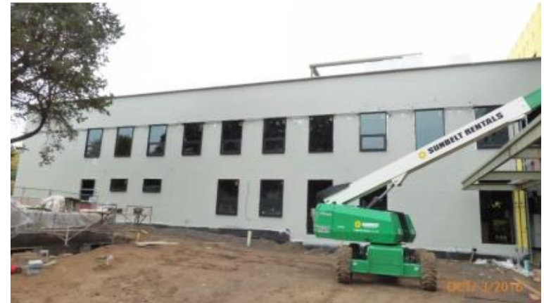
Exterior Windows – East side Sector A
